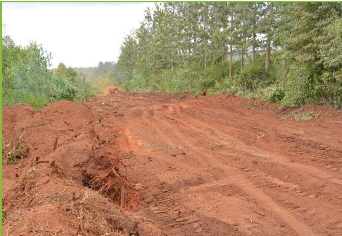
Ongoing road works
