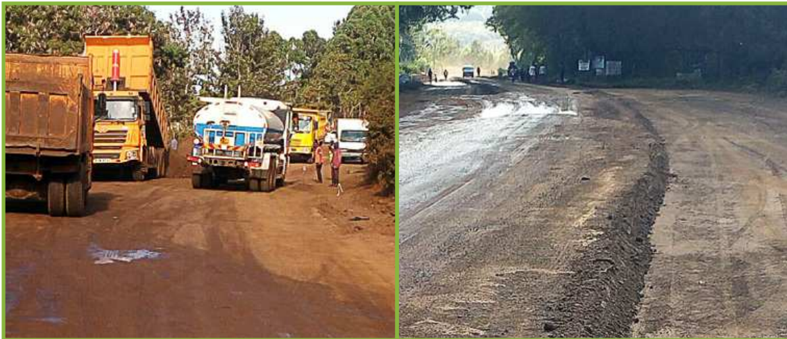
Ongoing road works on the Greater Eastern Bypass
